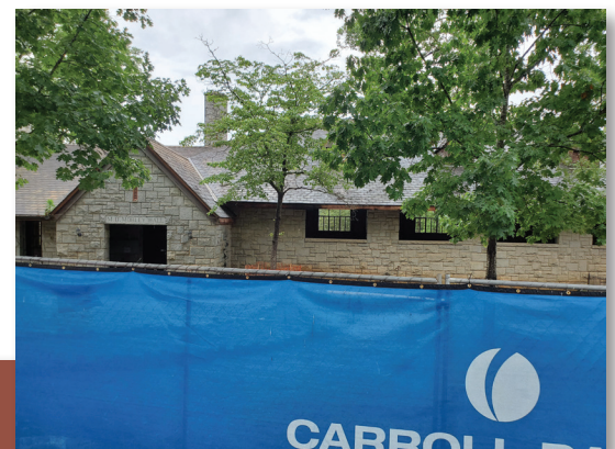
Renovation has begun on Mobley Hall
