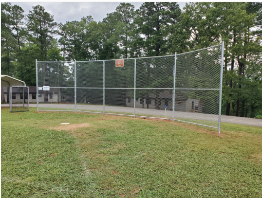
New Backstops have been added on the Softball Field
