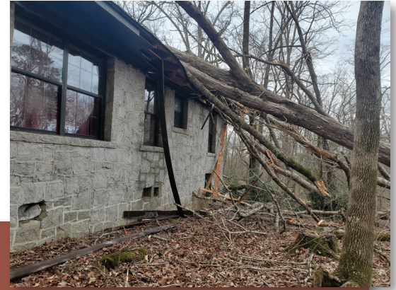
Cleanup and Cabin Repair after Tornadoes in January
